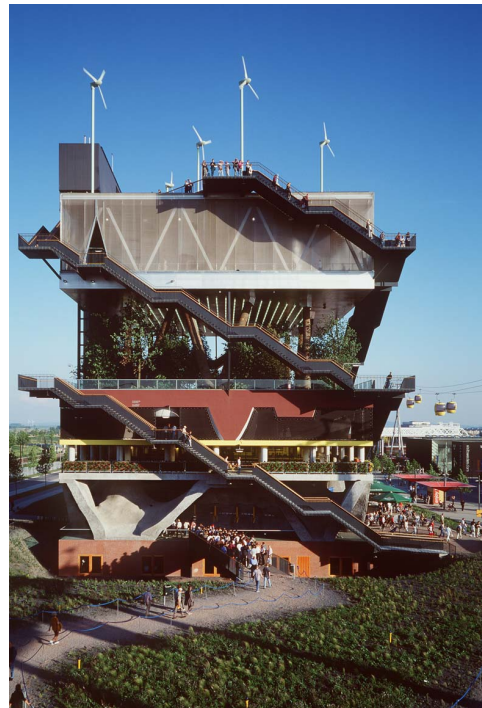
Figure 13, Opposing the current surroundings.
